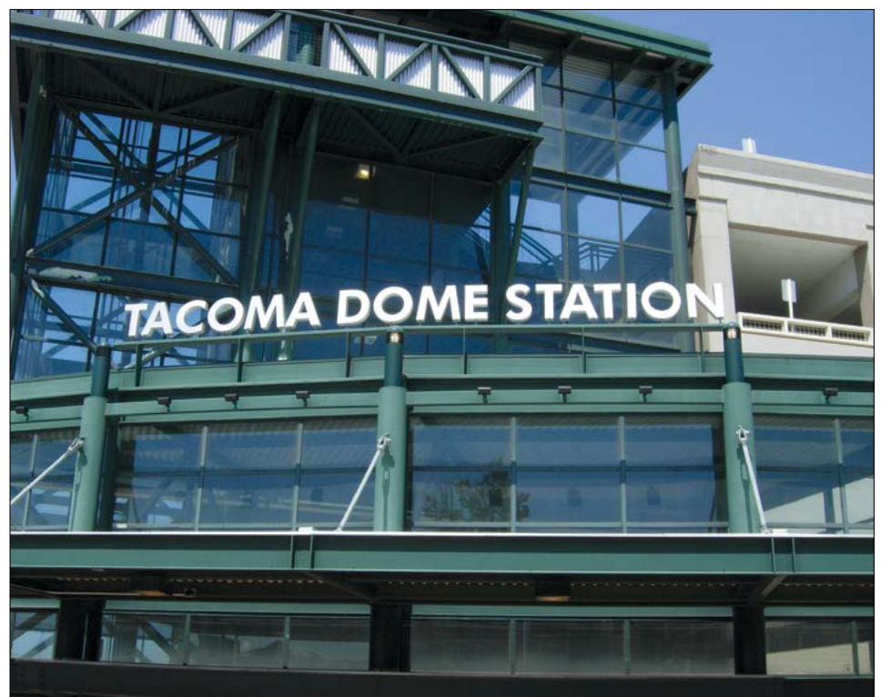
The Puget Sound Regional Council carried out subarea planning for the neighborhood around Tacoma’s Dome Station, once the southern terminus of the Sounder regional rail south line and home to the Tacoma Link.
