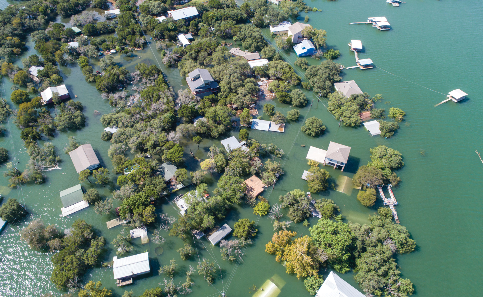
Climate change has increased the frequency and severity of natural disasters, including severe flooding events, which have also become increasingly costly.
