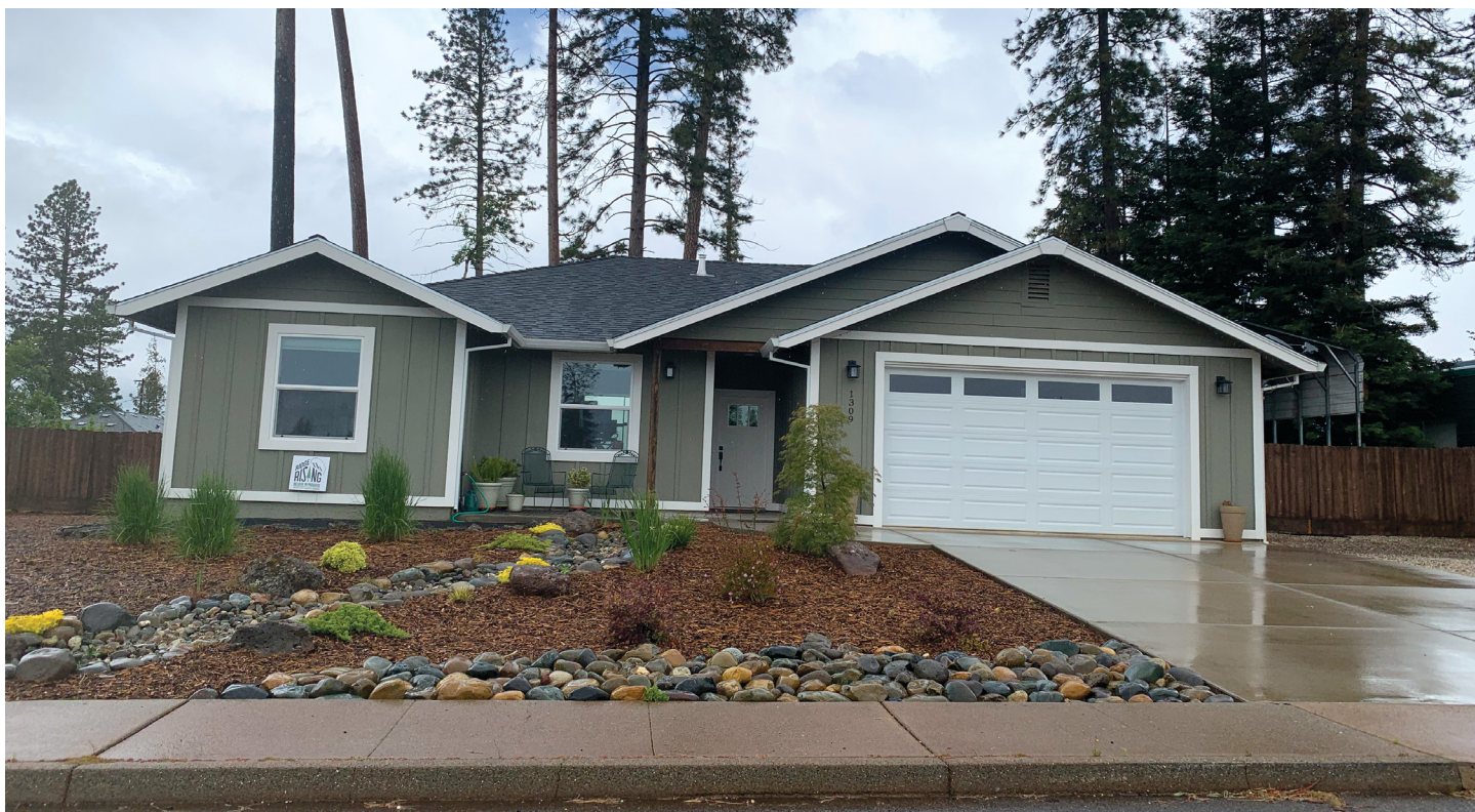
House designs such as the one above from the Rebuild Paradise Foundation's floor plan library use noncombustible building materials and follow local guidelines for defensible space surrounding the lot.
