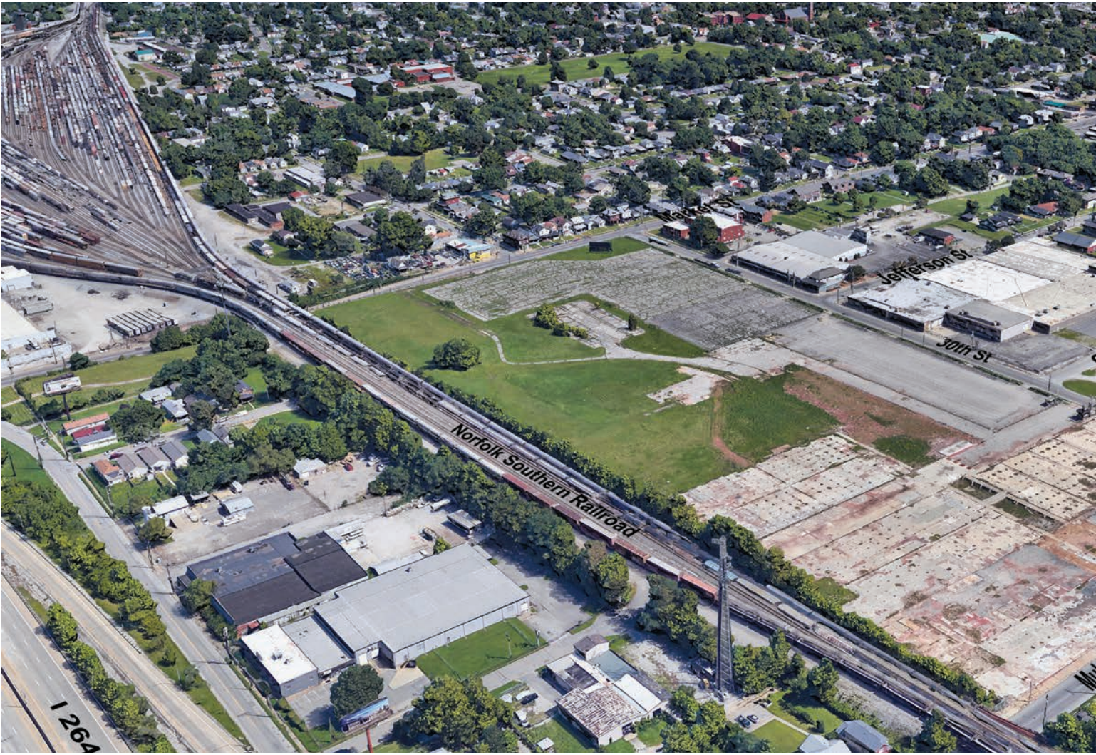
State and city governments, such as Louisville, Kentucky, have been proactive in marketing the investment potential of their Opportunity Zones.
