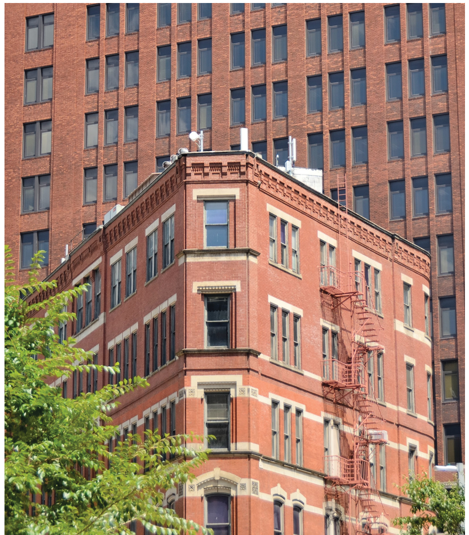
The Triangle Building is the first project selected for a PDCP loan to convert the property into 15 residential units above a ground-floor grocery store and café.
