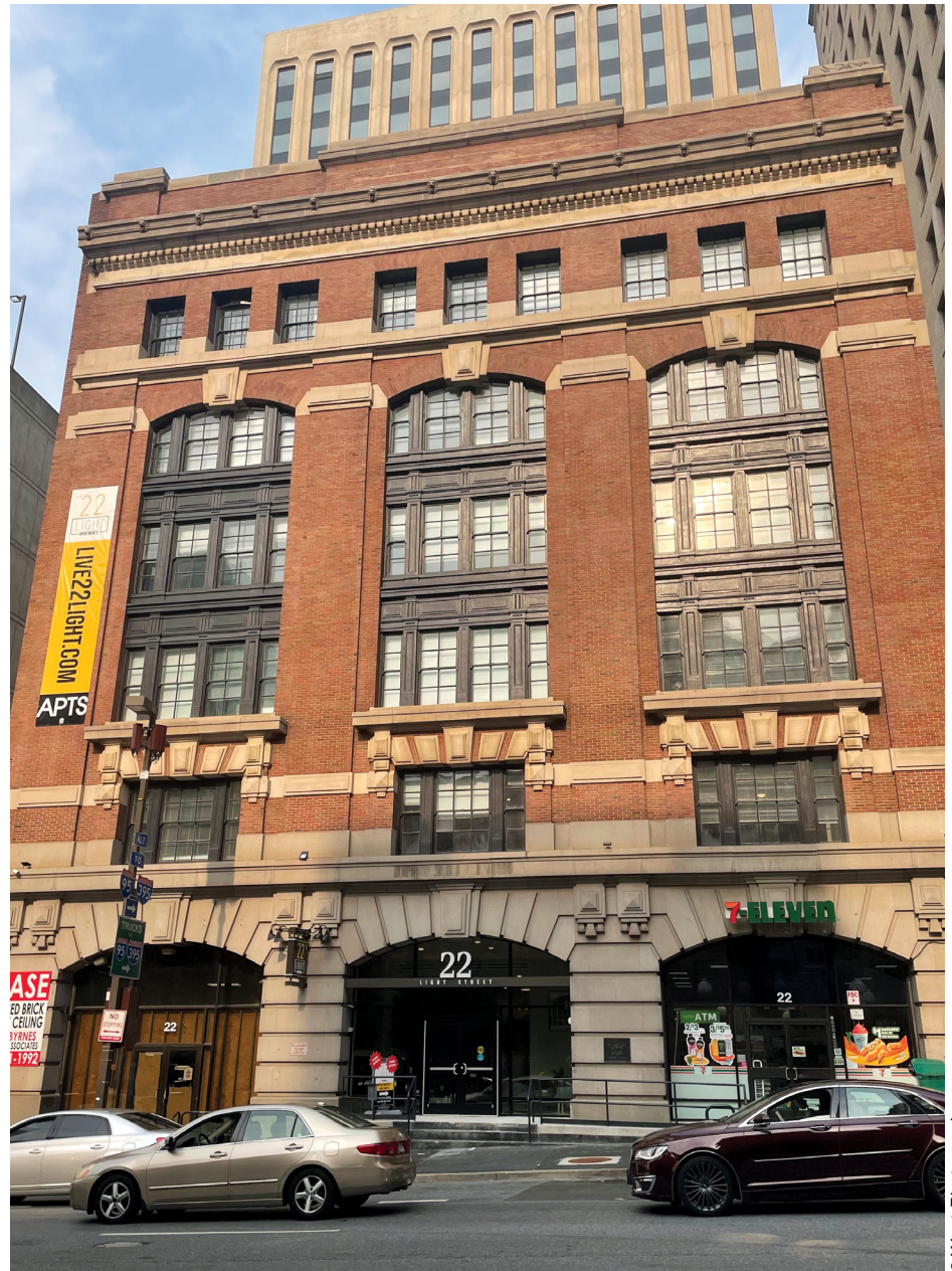
The conversion of the Lanahan building included preserving the windows and ornamental features of the building's historically significant front facade.
