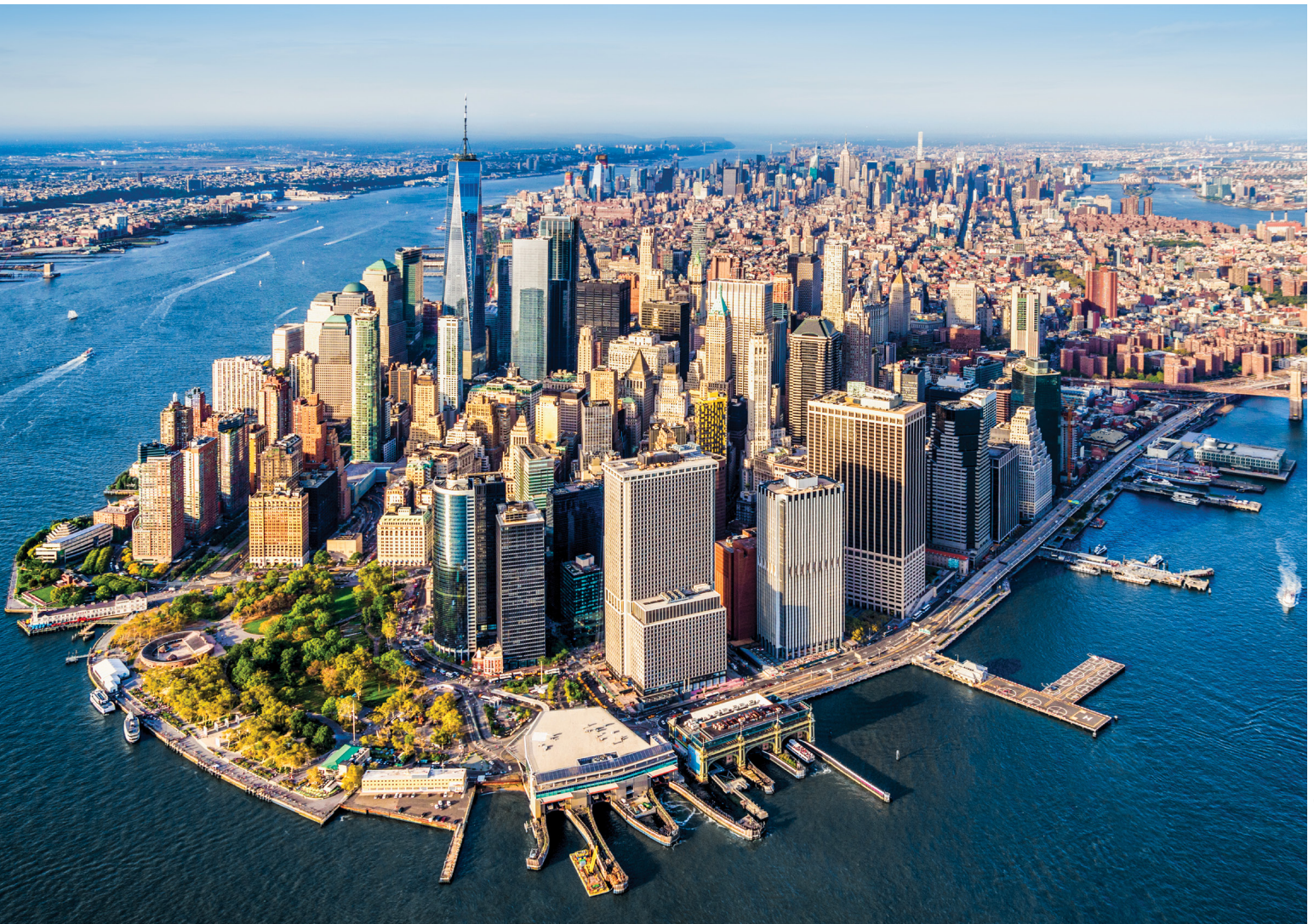
New York City implemented a property tax incentive program in the early 1990s to encourage office conversions as part of its plan to revitalize Lower Manhattan.
