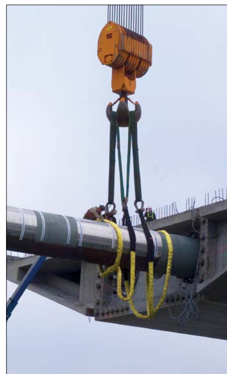
The newly reconstructed eastern span of the San Francisco-Oakland Bay Bridge uses hinge pipe beams that absorb seismic energy during an earthquake to protect the rest of the bridge. Damaged beams can be replaced following the earthquake.
