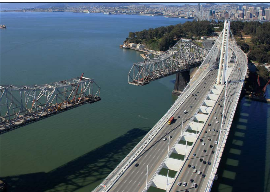
The newly reconstructed eastern span of the San Francisco-Oakland Bay Bridge uses hinge pipe beams that absorb seismic energy during an earthquake to protect the rest of the bridge. Damaged beams can be replaced following the earthquake.
