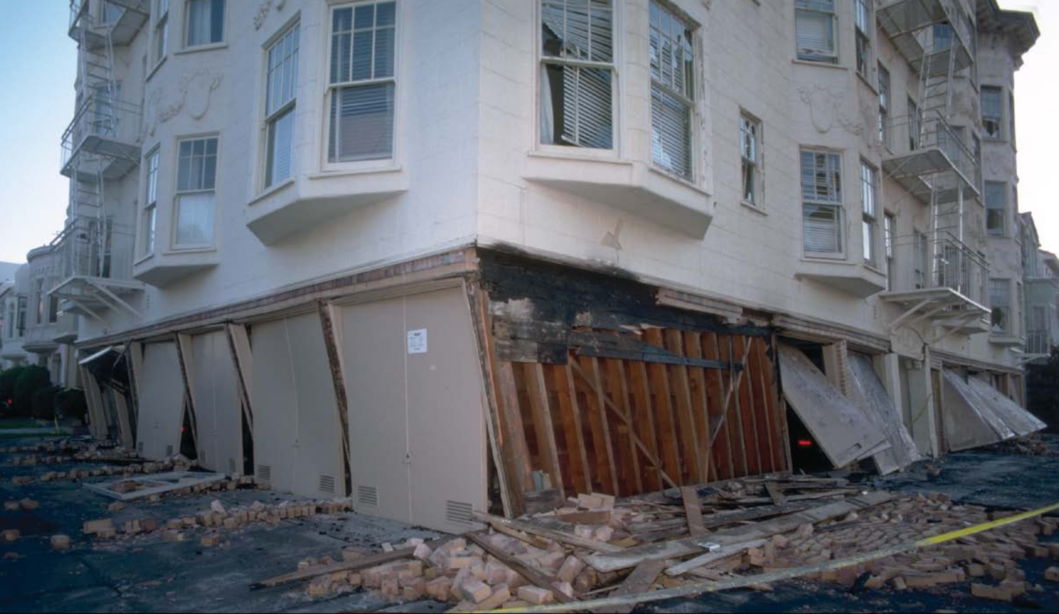
Soft story buildings are vulnerable to collapse because of their weakened ground floor support, often due to garage doors or large storefront windows.
