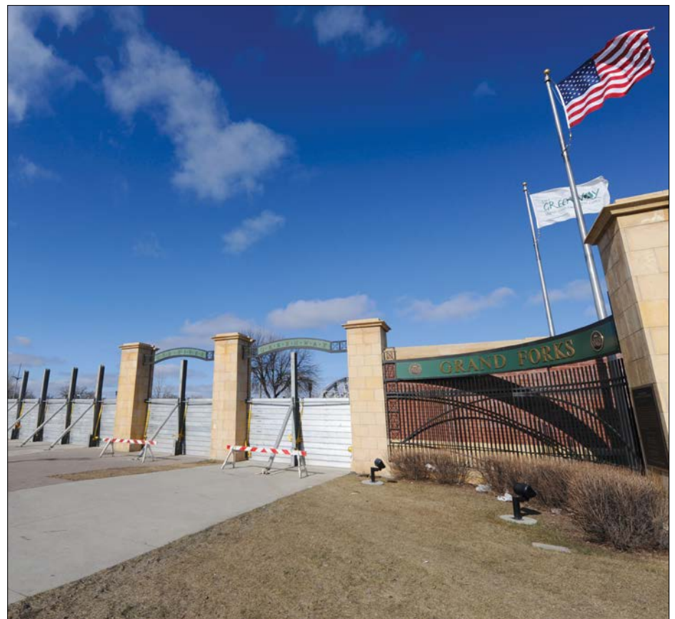
Floodgates help protect Grand Forks from rising water levels of the Red River.
