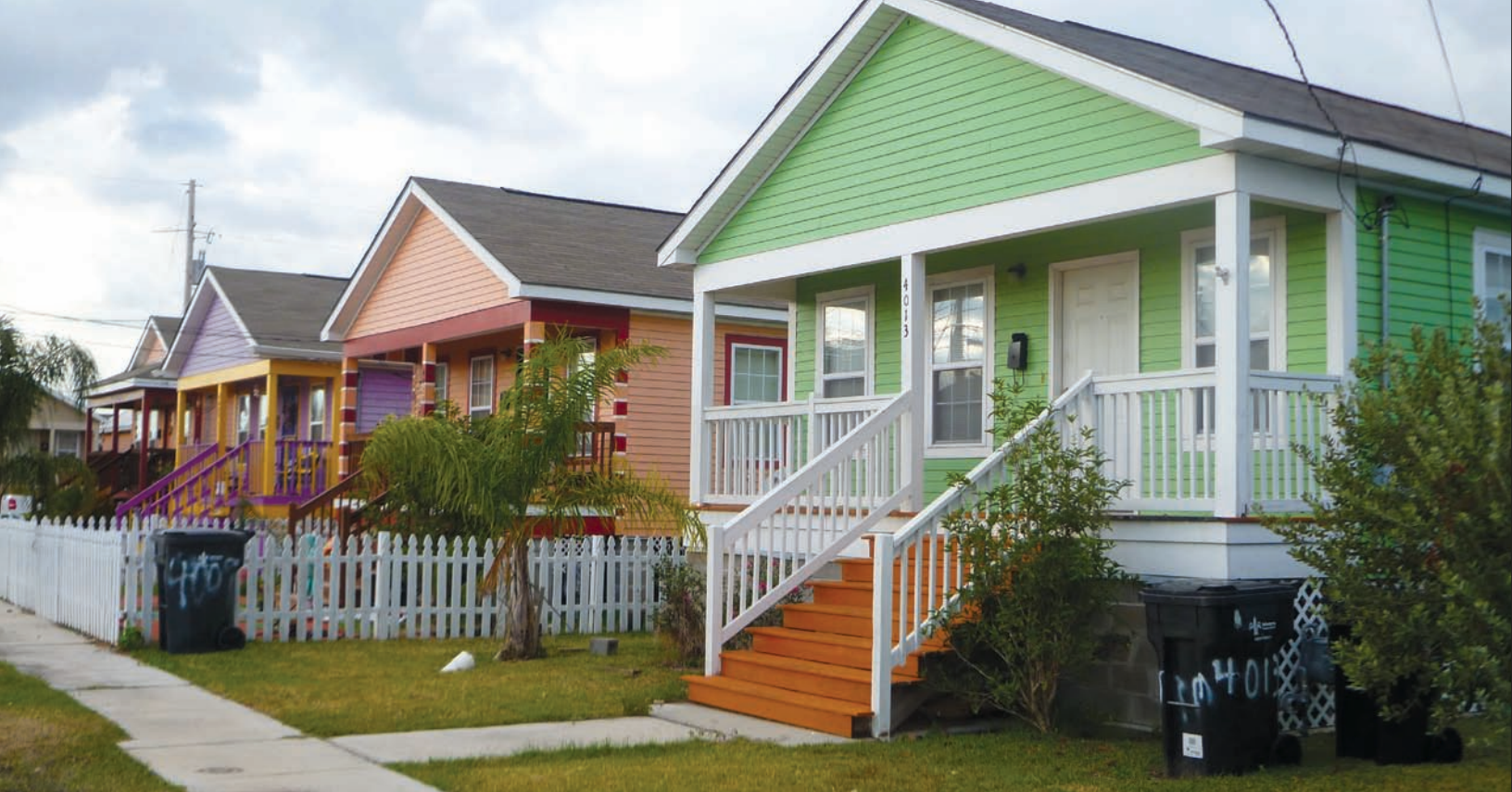
The Musicians' Village in the Upper Ninth Ward of New Orleans is part of the post-Katrina rebuilding effort that provides homes for musicians and other low-income families who were displaced by the disaster, while preserving the local culture.
