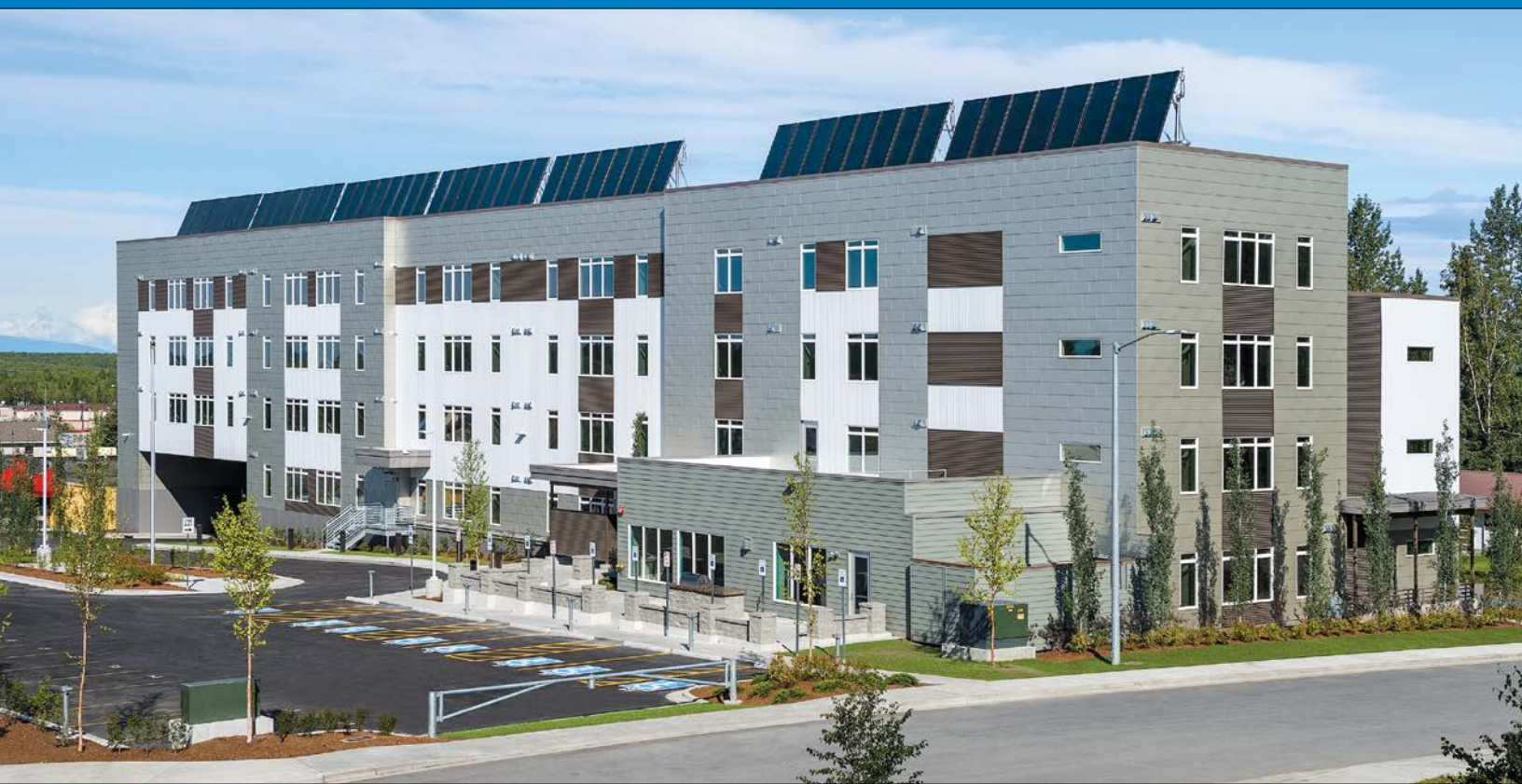
The Coronado Park Senior Village, part of a larger multigenerational, mixed-income community, helps support local business in Eagle River, Alaska by locating housing within walking distance of shops and services.
