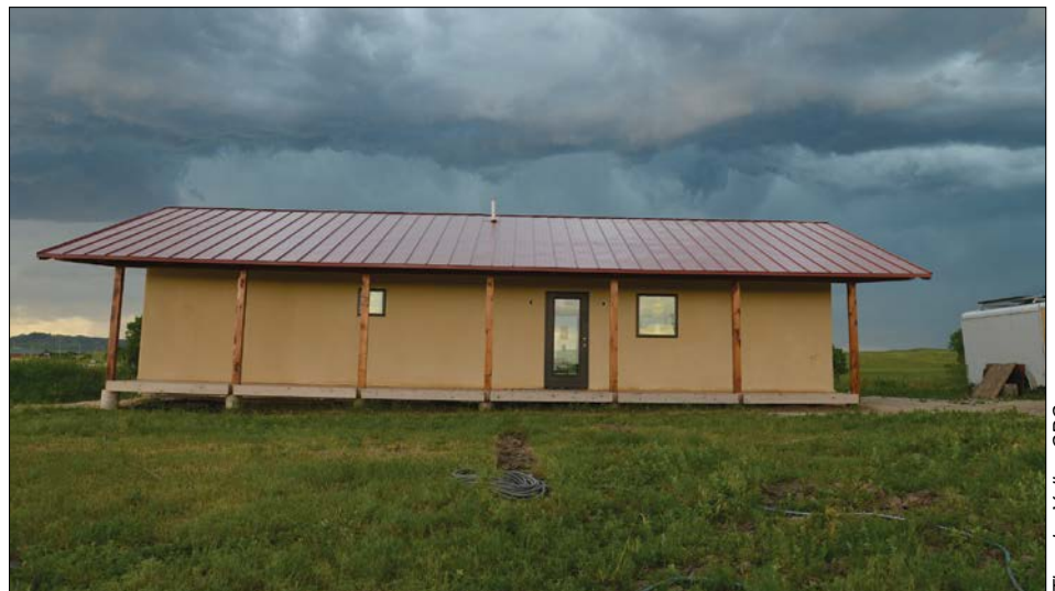
In partnership with the University of Colorado Boulder's Native American Sustainable Housing Initiative, the Thunder Valley Community Development Corporation is constructing energy-efficient, sustainable housing like the straw-bale design pictured above.
