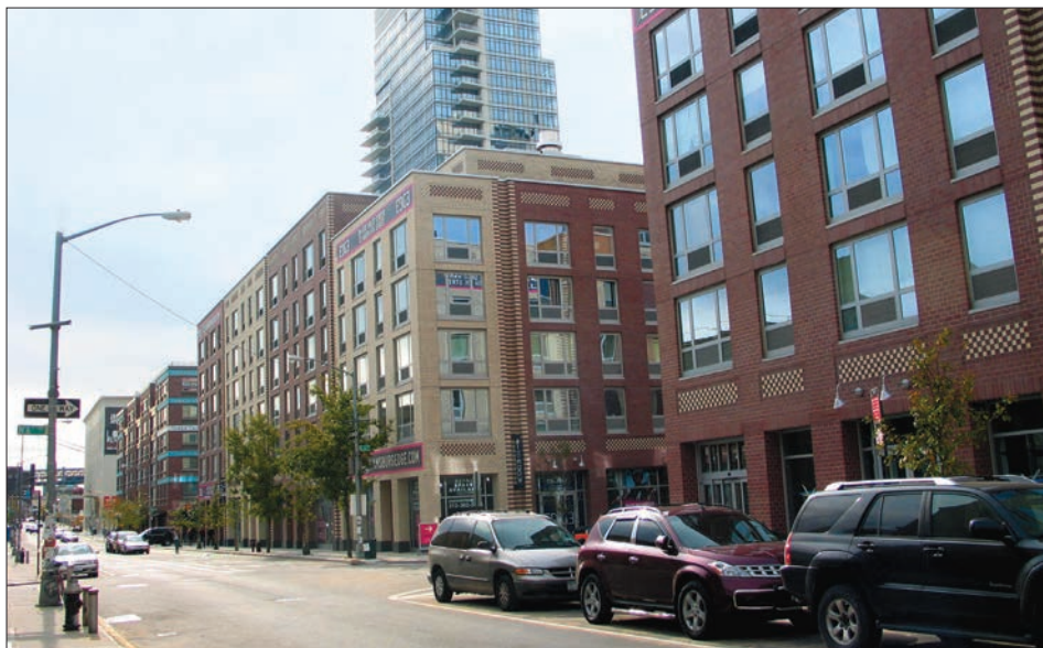
Palmer’s Dock and Edge Community Apartments are the affordable housing component of the larger Northside Piers and Edge developments along the Brooklyn waterfront. Both projects, located within the Greenpoint-Williamsburg inclusionary housing designated area, received density bonuses and tax abatements from the city in exchange for providing affordable housing.
