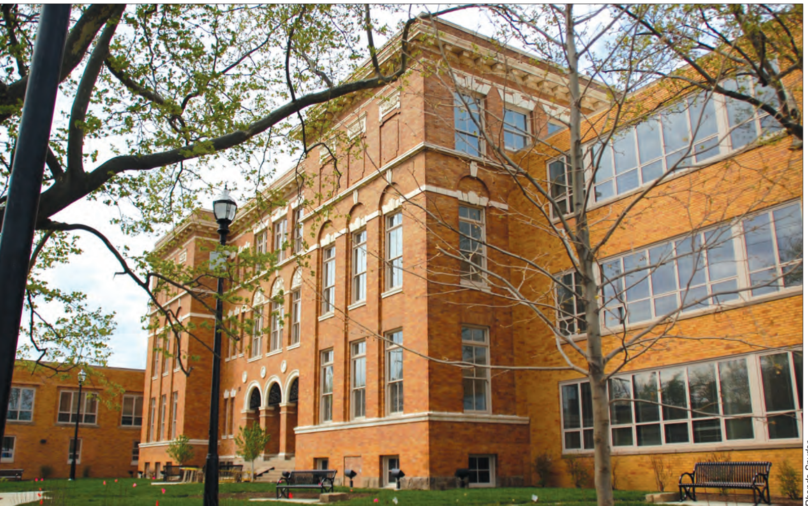
Part of financing for the rehabilitation of Doan Classroom Apartments in Cleveland, Ohio came from the Ohio Preservation Loan Fund. Listed on the National Register of Historic Places, this building offers 45 affordable senior housing units.
