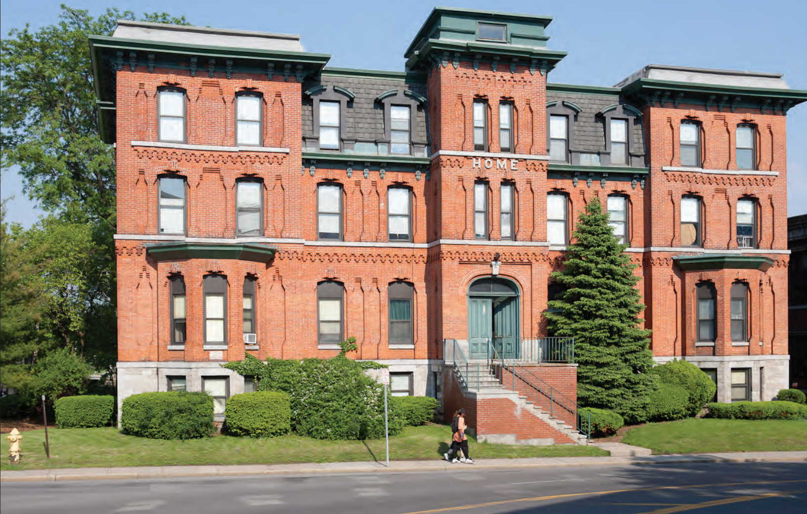
The Moses Dewitt Redevelopment project in Syracuse, New York will rehabilitate and preserve 37 apartments for very low-income seniors.
