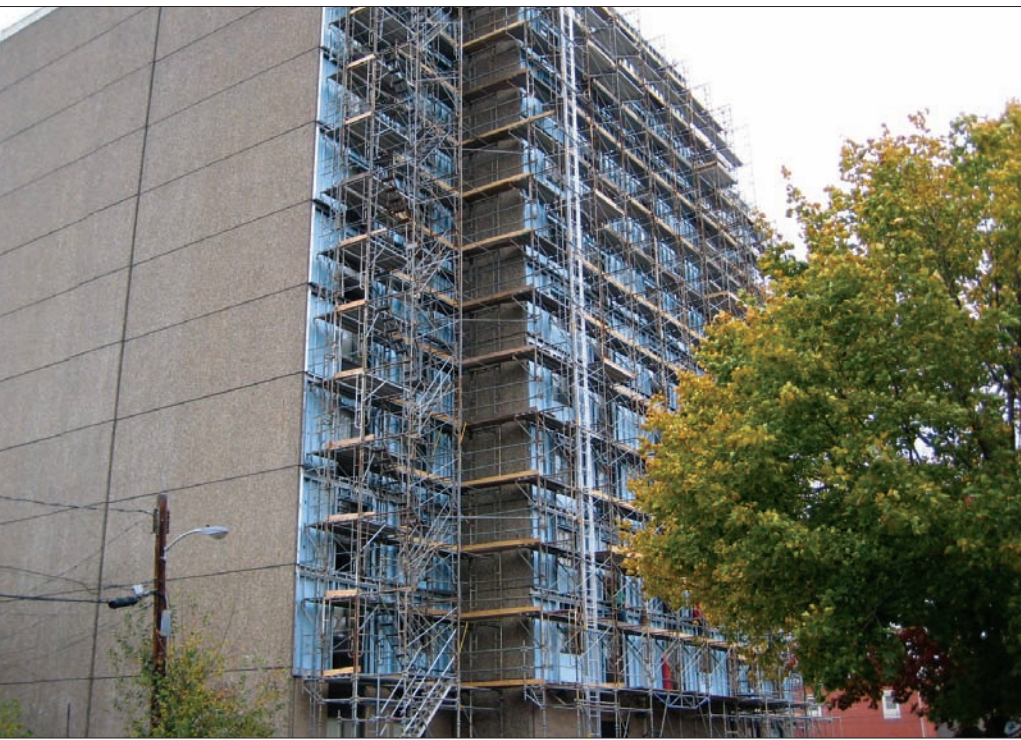
Green retrofitting of multifamily housing built prior to 1990 — such as this building that is having insulation added to exterior walls and its windows replaced — can mean substantial savings in energy consumption/costs.
